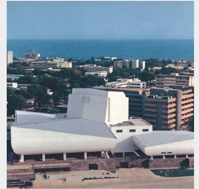
Manama - BAHRAIN Nawab Extension Project
