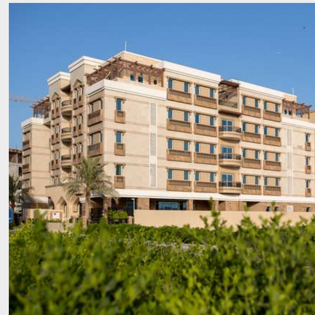
Doha - QATAR Fox Hill Project
