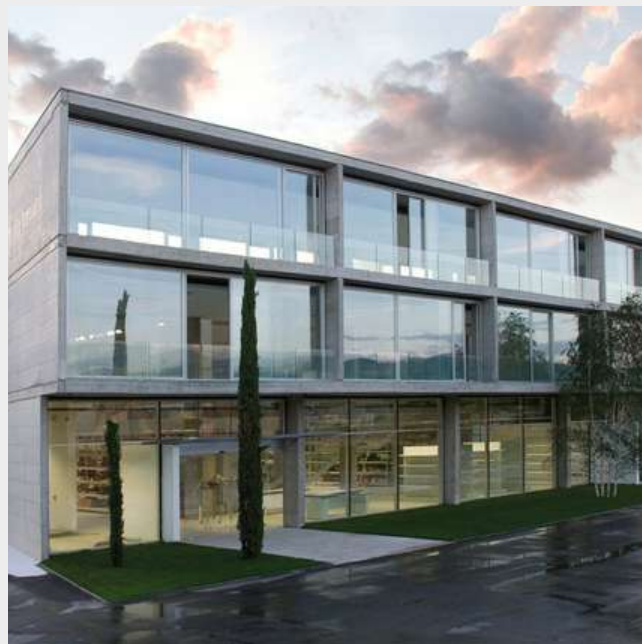
Niksic - MONTENEGRO Neckom Office Project
