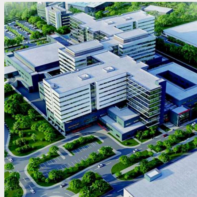
Astana - KAZAKHSTAN Nur Sultan Hospital Project
